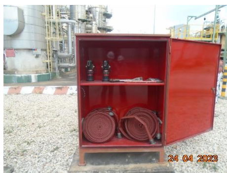
Fire Hose Box and Nozzle
