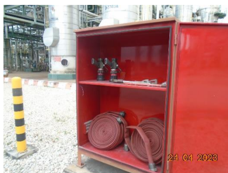
Fire Hose Box and Nozzle
