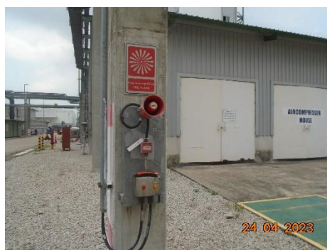
Fire Alarm Manual Station
