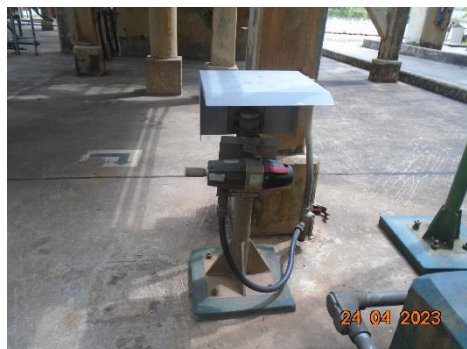
Combustion Gas Detector
