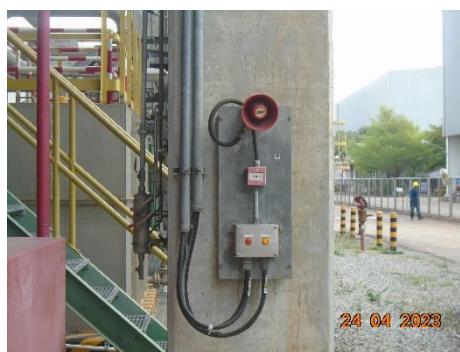
Fire Alarm Manual Station
